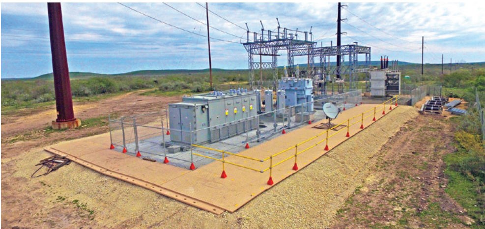
Equipotential zone utilizing our fully integrated mat system for a Temporary Substation.
