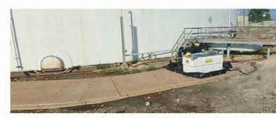
**DURA-BASE**° Turning Mat provides a 10 degree change in direction to the path of a single lane DURA-BASE Road.
