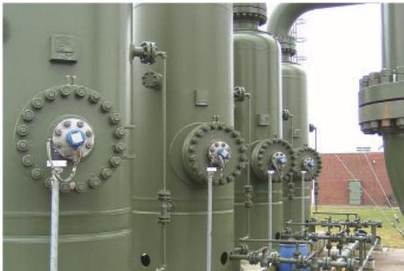
A typical compressor station consists of an inlet scrubber to collect liquids and slugs that may have formed in the gas pipeline. The scrubber consists of a primary section where liquids and solid parts are separated from the gas stream
