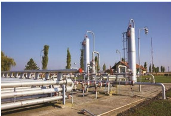
Separating the hydrocarbons and fluids from pure natural gas produces pipeline quality dry natural gas. Absorption and cryogenic expander are the two methods used for removal of natural gas liquids.
