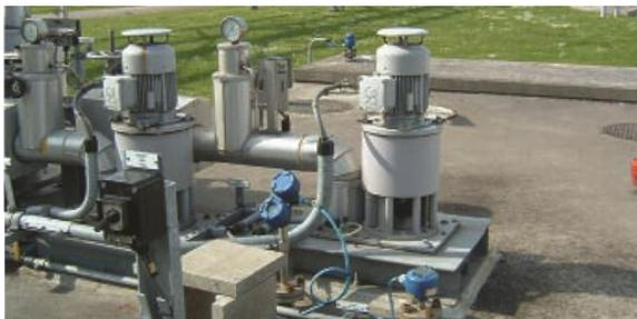
Liquid waste from compressor station scrubbers & filters can be condensates or hydrocarbons from the natural gas. The wastes are collected in one or several tanks depending on the size of the remote station. Waste tank trucks are scheduled for emptying operations that are classified as hazardous materials.
